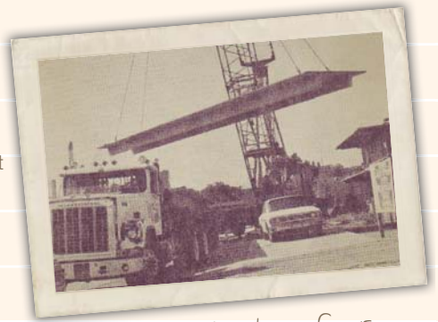
The construction of our adoptions building
